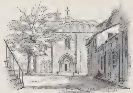
No. 40.—Façade of Cadouin.
